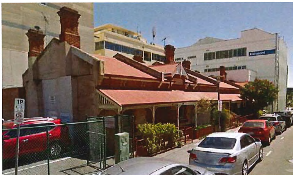
Figure 7: Cottages, Gray Street, West Side, 1969 (No. 25 and 21, in foreground, later demolished)
