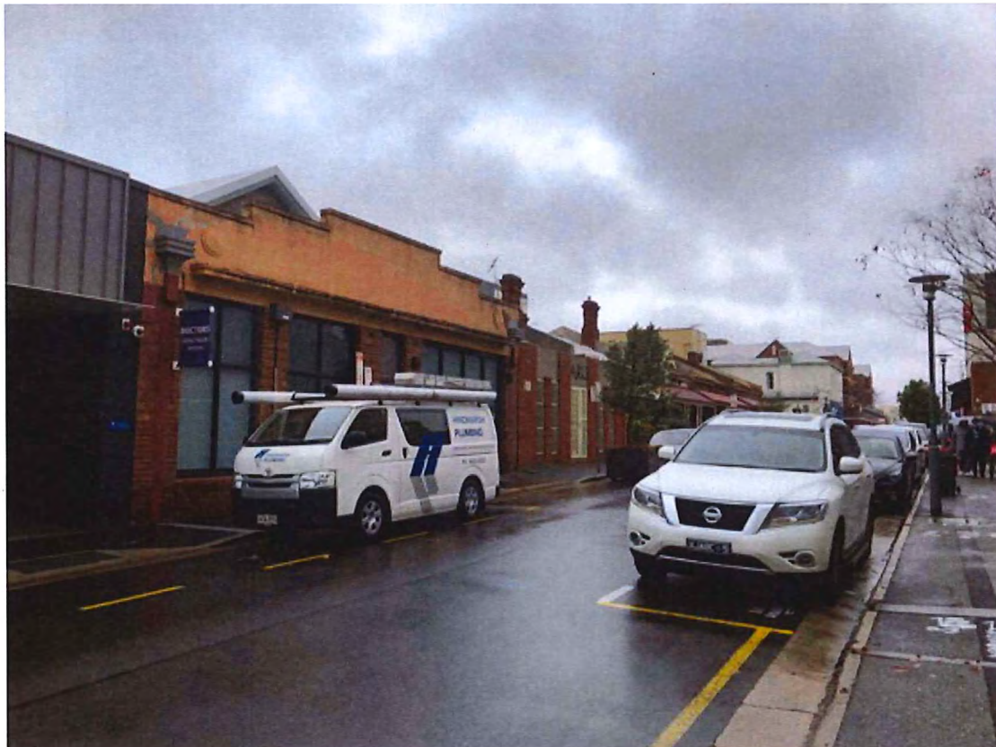
Figure 5: View from the Subject Site looking South East along Gray Street Source: Flightpath Architects, 2019
