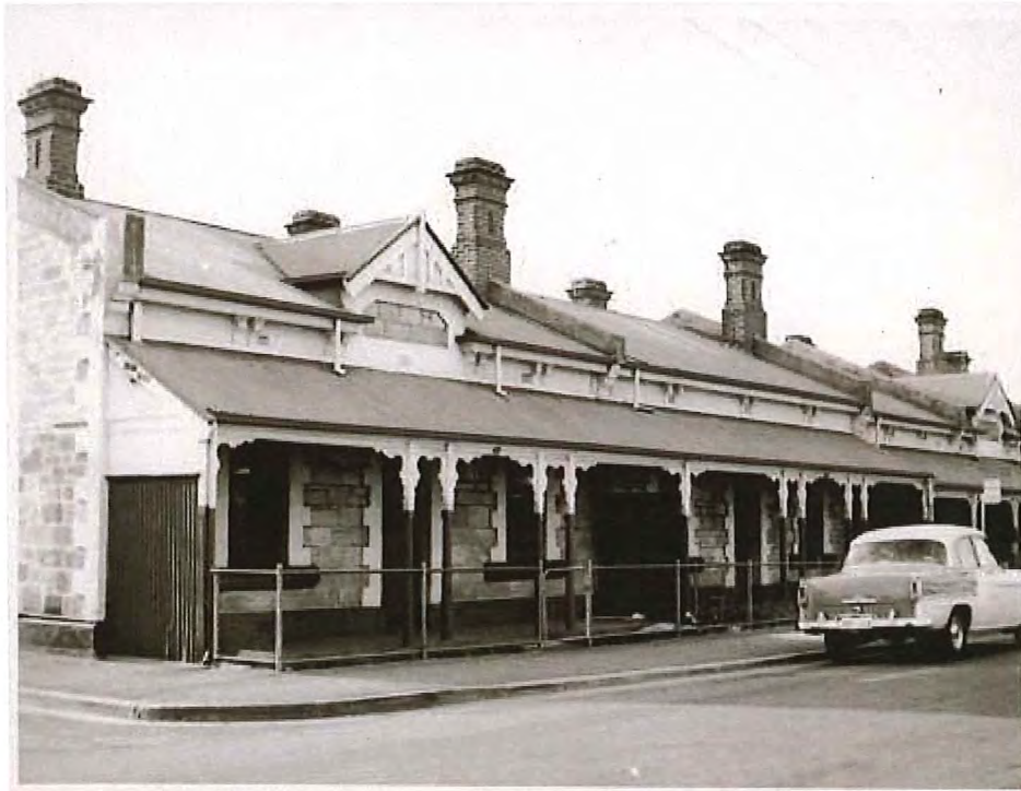
Figure 6: Cottages, Gray Street, West Side, 1969 (No. 25 and 21, in foreground, later demolished)
